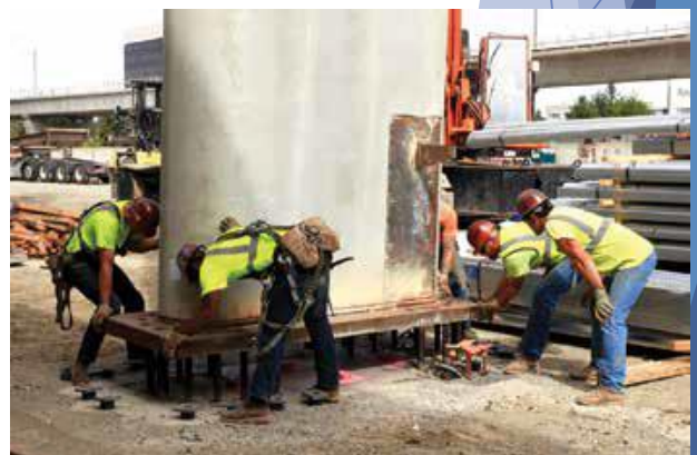
Wall units were handled using rigging inserts placed on the manually finished side, and they were anchored to foundations using cast-in-place anchor rods
