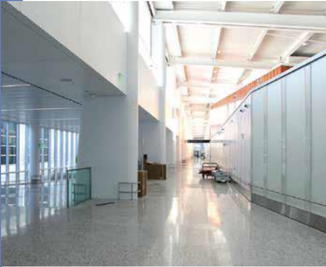
A view of the walls as the project nears completion
