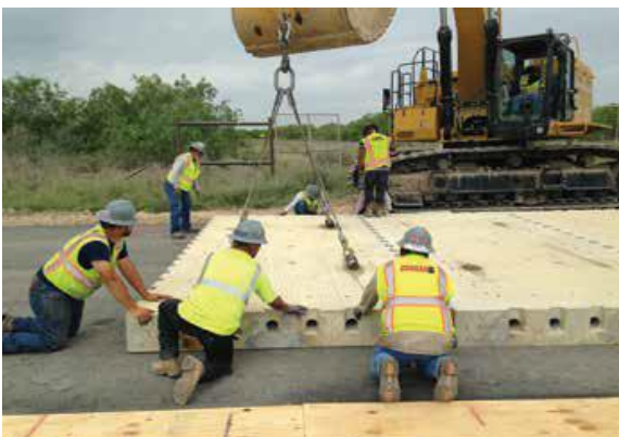
Fig. 9: A panel being placed on the HMA base
