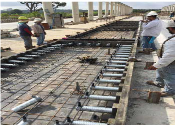
Fig. 7: Panel formwork within a prestressing bed
