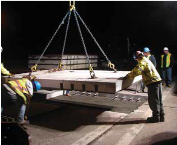
Fig. 1: A PCP repair is installed to restore an isolated pavement joint
