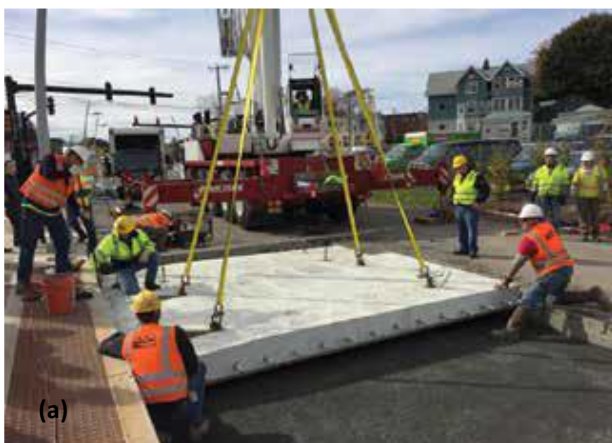
Fig. 4: A typical precast panel used for rehabilitation of two Ctransit bus pads: (a) dowel bars embedded at one transverse side; and (b) dowel bar slots along the opposite side
