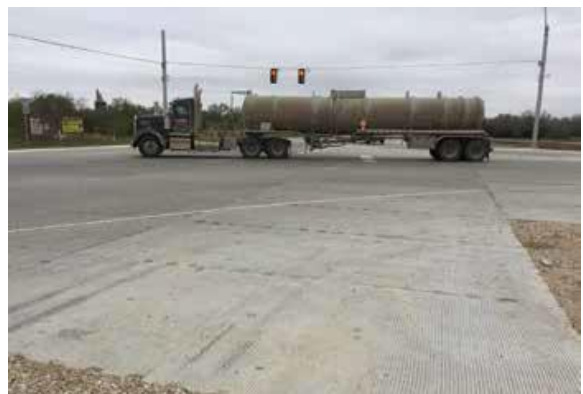
Fig. 10: Completed intersection in use (view from SH 97)
