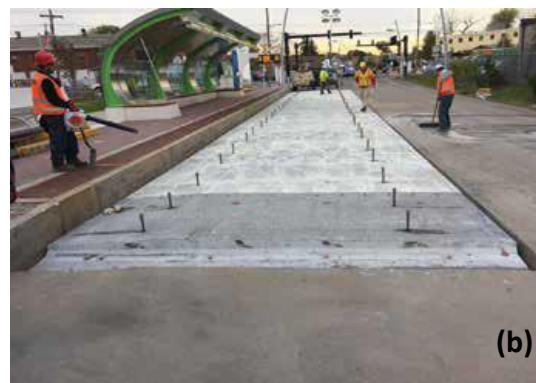
Fig. 5: The north bus pad rehabilitation: (a) placement of the first panel; (b) placed panels with leveling lifts engaged; and (c) in operation
