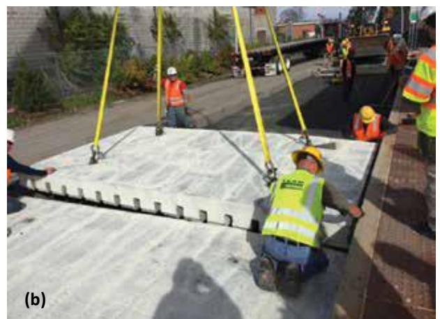
Fig. 4: A typical precast panel used for rehabilitation of two Ctransit bus pads: (a) dowel bars embedded at one transverse side; and (b) dowel bar slots along the opposite side
