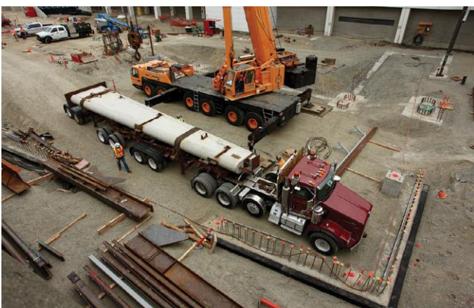
Walls weighed from 45 to 93.5 tons (41 to 85 tonnes) and were delivered using special transports
