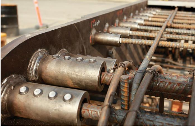
Shear-bolt couplers were welded to steel embed plates to connect longitudinal bars at the base of each wall
