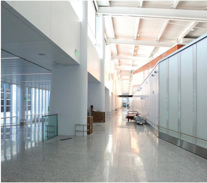
A view of the walls as the project nears completion
