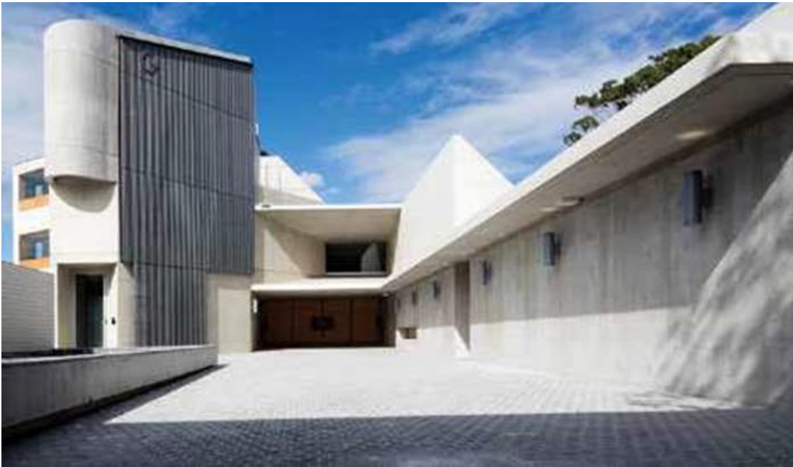
Fig. 1: Punchbowl Mosque, Sydney, Australia, with main entry doors facing the street and a single minaret adjacent to the entry (left) (photo by Brett Boardman, courtesy of Candalepas Associates)
