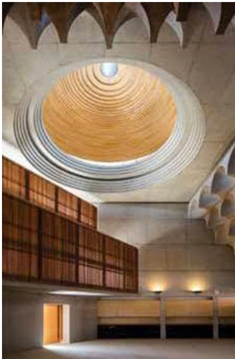
Fig. 2: A view from the floor of the main prayer hall, showing the stepped soffit of the concrete ring beam and rows of quarter- sphere muqarnas. Since this photo was taken, Turkish and Iranian calligraphers have inscribed the smooth and seamless concrete surfaces of the minidomes with the 99 names of Allah in gold calligraphy (photo by Brett Boardman, courtesy of Candalepas Associates).
