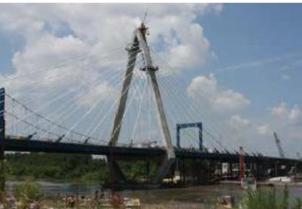
Christopher S. Bond Bridge project credits: MoDOT, Owner; Parsons Corp., Engineer; Paseo Corridor Constructors (a partnership of Massman Construction Co, Clarkson Construction Co, and Kiewit Construction Co), Contractor; and Fordyce Concrete, A Division of Ashgrove Materials Corp, Concrete Supplier
