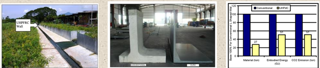
Fig. 8. (a) 90m monsoon drain using retaining wall, (b) comparison of conventional precast retaining wall with ultra-light weight UHPC retaining wall, and (c) EIC comparison with conventional retaining wall [19].
