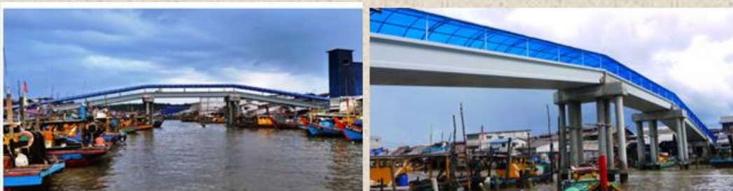
Fig. 5. Malaysia’s first multi-span motorcycle-pedestrian bridge crossing Sg Sangga Besar, Perak [17].
