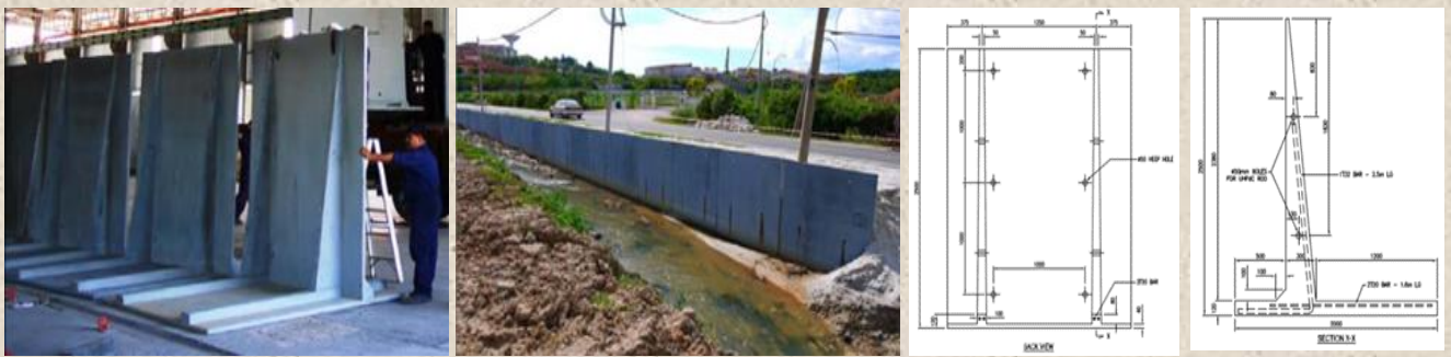
Fig. 9. (a) Prototype of UHPC retaining wall, (b) 76 m long retaining wall at Jalan Kota Bahru, Gopeng, (c) Drawing detail of retaining wall [7]
