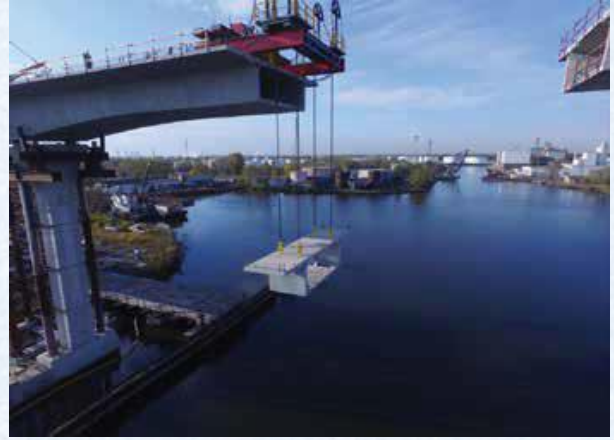
Engineered Rigging chose Enerpac strand jack technology to complete the span over the canal
