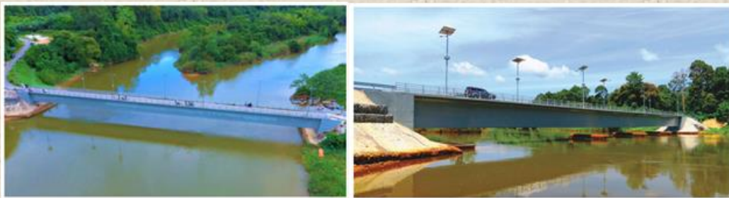
Fig. 6. World’s longest UHPC single-span bridge at Batu 6, Gerik, Perak [18].
