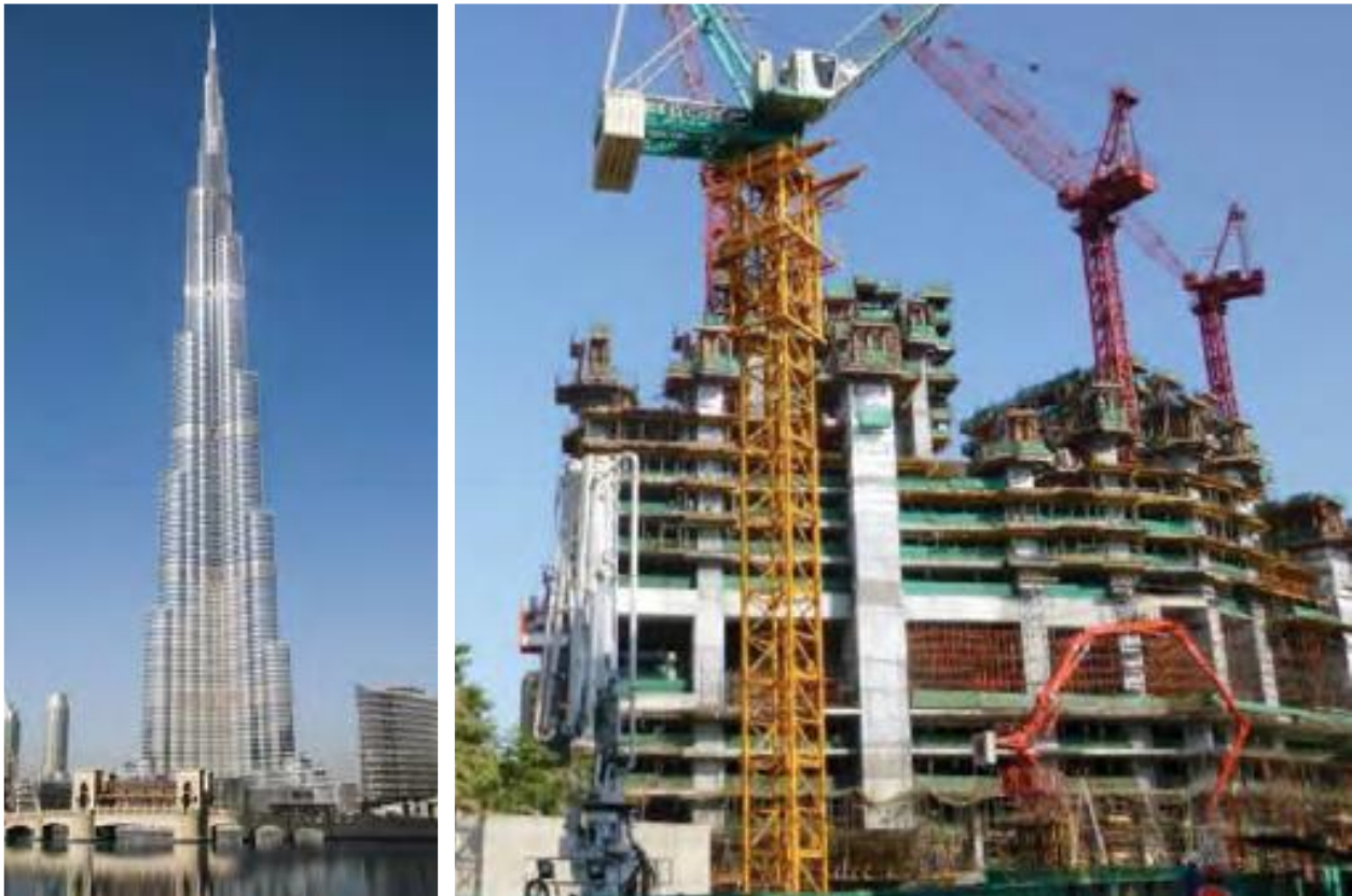
Fig. 3: Tallest high-rise buildings: (a) Burj Khalifa; and (b) construction of the Worli Project (photo courtesy of Pierre-Claude Aïtcin)
