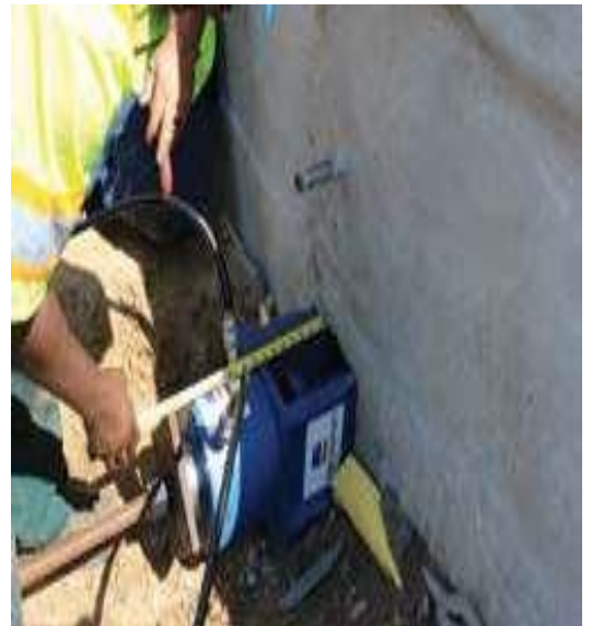
Fig. 11: A worker checks tendon extension during the tensioning operation
