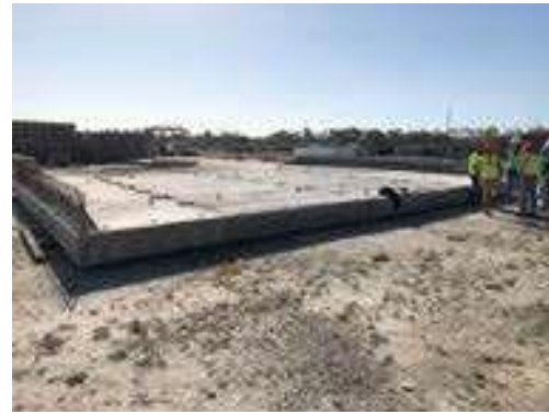
Fig. 4: Panel fit-up was verified at the precast plant on March 27, 2018.
