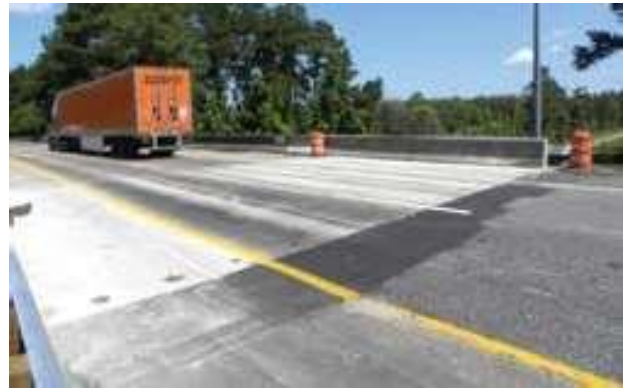
Fig. 12: Completed bridge approach slab
