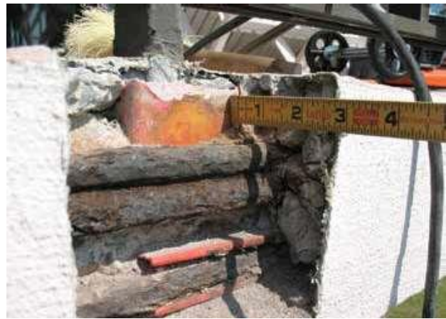
Fig. 2: Example of test excavation during 2007 assessment
