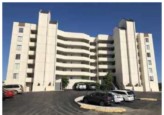
Fig. 1: Sound of Sea II Condominiums. (a) viewed from the beach; and (b) viewed from the parking lot in 2019 (more than 10 years after repairs).
