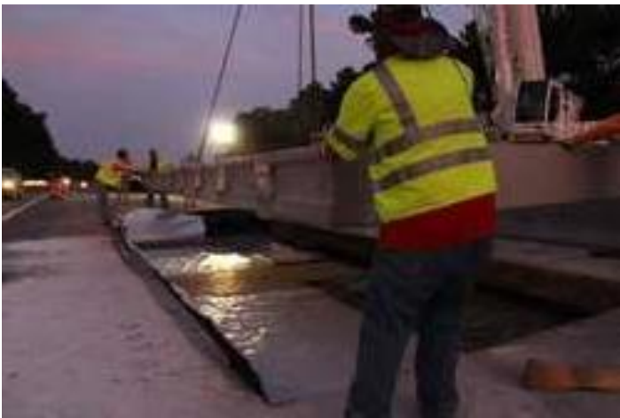
Fig. 8: Panel installation: (a) Panel A; and (b) Panel C
