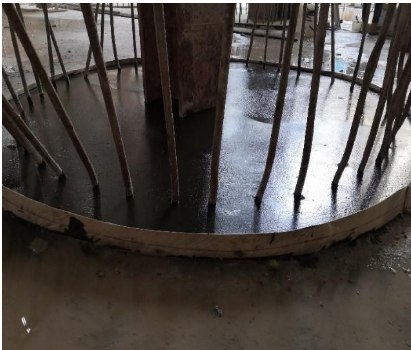
Photo 2: Pile head treated with epoxy grout
