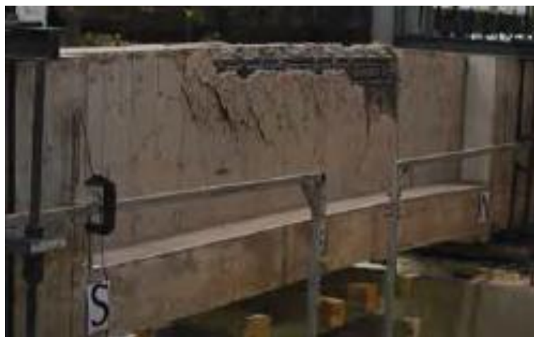
Fig. 7: Splice failure in test beam
