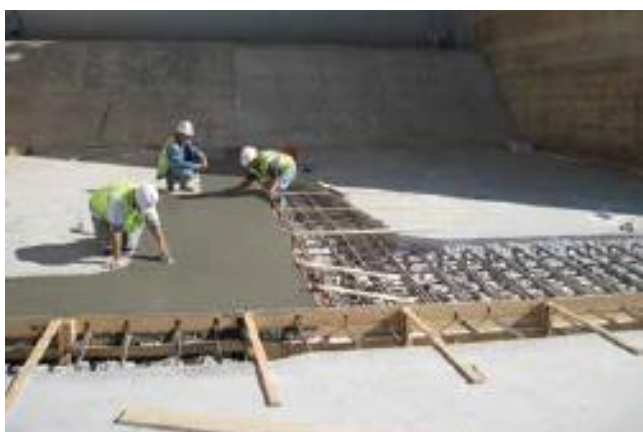
Fig. 3: Placing concrete back to the original lines and grades
