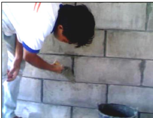
Figure 1. Using LFC blocks in a Malaysia
