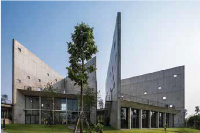
Fig. 2: Concrete and glass are the main components of the building's structure and façade
