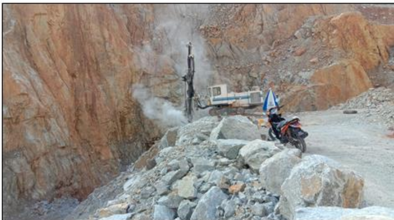
Rock Drilling & Blasting Work
