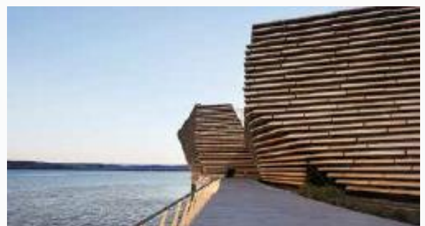
Fig. 3: The striated building façade invokes images of the Scottish coastline cliffs (photo courtesy of HUFTON + CROW)
