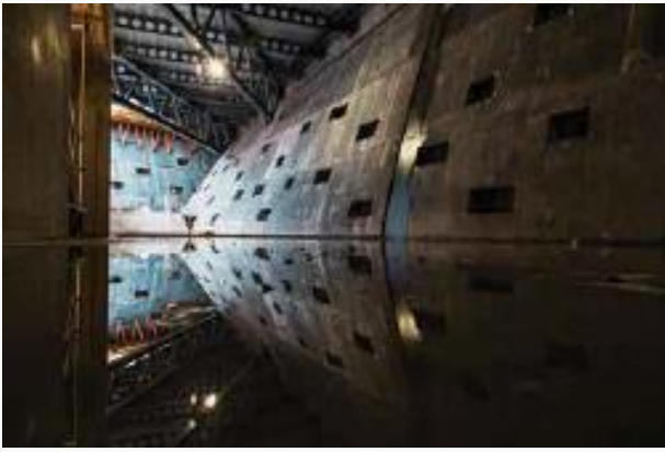
Fig. 7: The building is a hybrid structure with external walls, internal shear walls, and main cores constructed using reinforced concrete, and the first floor, second floor, and roof constructed using structural steelwork
