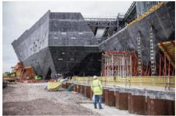
Fig. 6: Two inverted pyramids are separate up to the second floor, at which point they are joined
