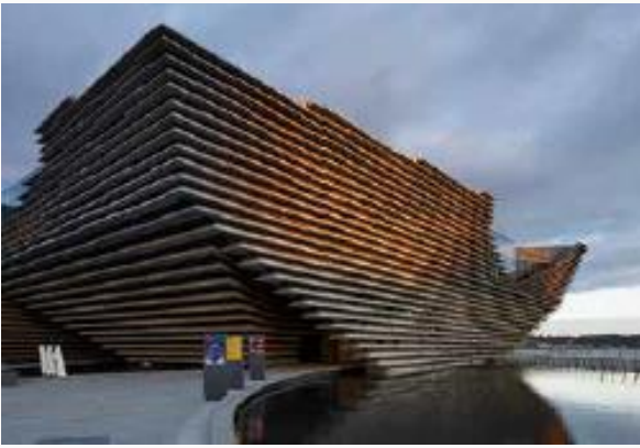
Fig. 10: The cliff face appearance of the building's exterior was executed with 2429 precast concrete panels
