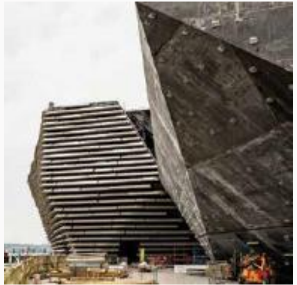
Fig. 9: Façade walls made of dark and smooth concrete
