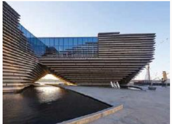
Fig. 2: The building has the form of two inverted pyramids (photo courtesy of HUFTON + CROW)
