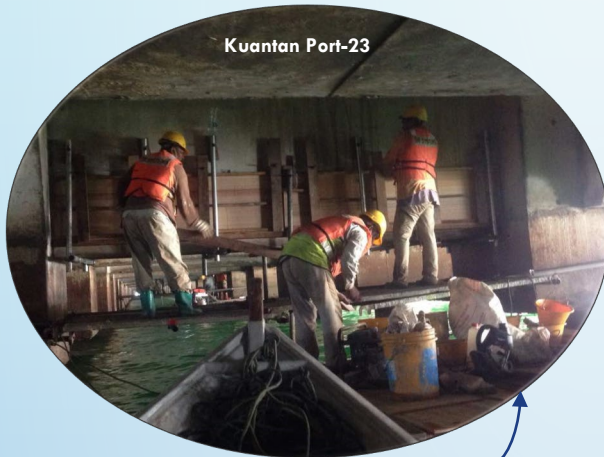
Preparing formwork to under wharf for concrete repair.
