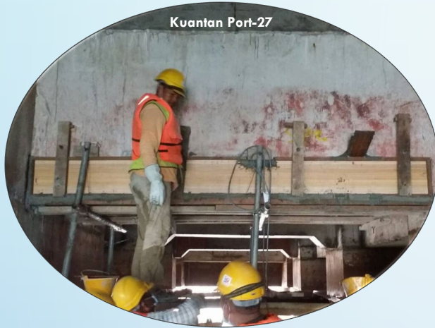
After application of Mapefill MC 06
