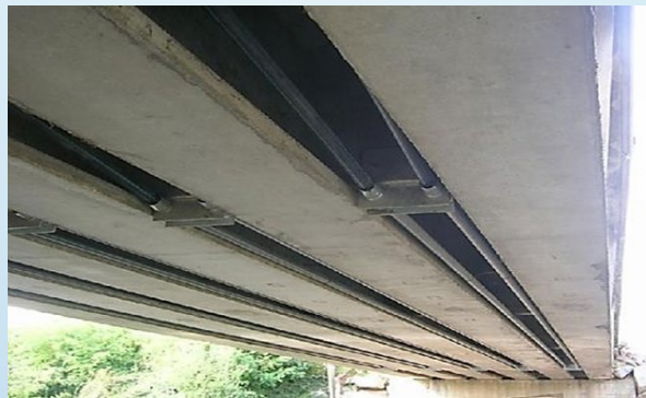
Fig. 5. Real life strengthened bridge (EPT Technique)
