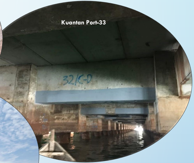
Completed works of refurbishment of Kuantan Port
