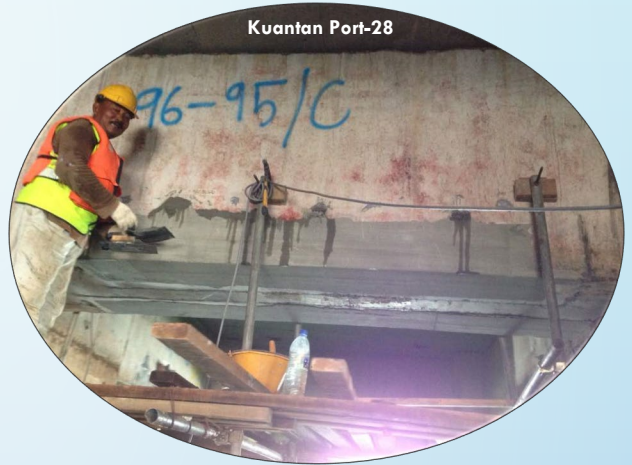
Continue with the application of Planitop G40 SP
