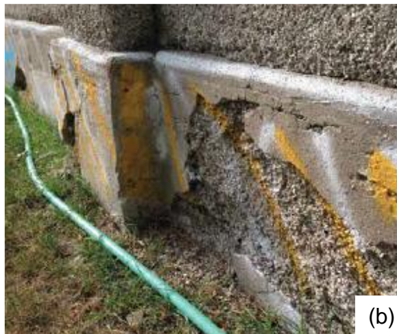
Fig. 2: Perimeter walls at St. Boniface Cemetery, Chicago, IL: (a) a general view; and (b) close-up of the deterioration of the 1/8 in. (3 mm) thick mortar coating on the porous concrete foundation
