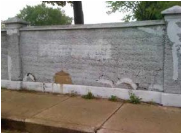
Fig. 7: Repairs made using a nonpervious mortar mixture are unattractive, and they could be accelerating corrosion damage by clogging the open textured matrix and reducing drainage of any accumulated water within the wall
