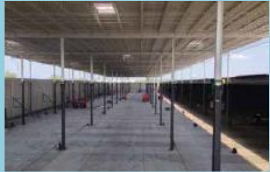
An example of capturing unused air space to enlarge an industrial facility (photo courtesy of John J. Bernauer, EZ Riser Roof Raising Services)
