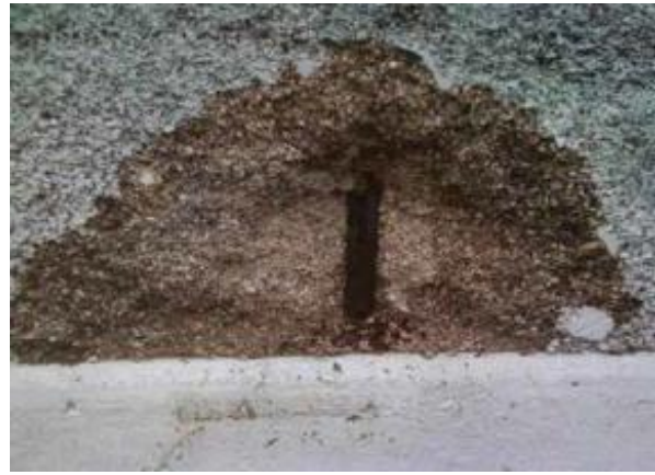
Fig. 7: Repairs made using a nonpervious mortar mixture are unattractive, and they could be accelerating corrosion damage by clogging the open textured matrix and reducing drainage of any accumulated water within the wall
