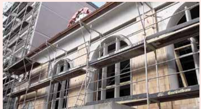
The window frames near completion. After the joints were mortared, the frames were painted to complete the facade restoration
