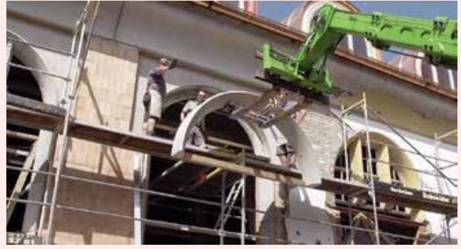
Concrete elements were assembled and installed at the project site
