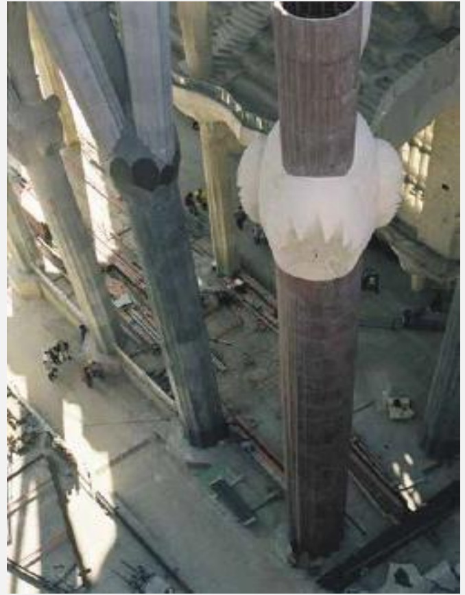
Fig. 6: Stone or precast concrete exterior “drums” were used to form the trunks and branches with reinforced concrete cores (© Fundació Junta Constructora del Temple de la Sagrada Família)
