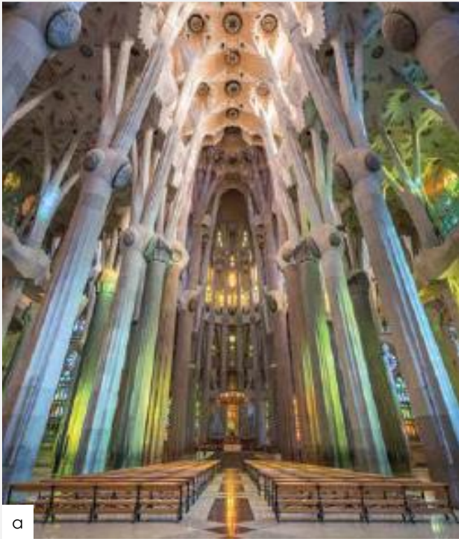
Fig. 4: The interior of the cathedral is a celebration of light: (a) Tree-like columns and their “branches” line the main nave, seen here looking toward the apse. Four types of columns have been constructed: columns on each of the four corners of the crossing support the Jesus Christ tower and partially the weight of four Evangelist towers; columns that bear the main load of the four Evangelist towers; columns in the apse and naves; and columns that separate the side naves from the main nave; and (b) The longitudinal nave on the Nativity façade side of Sagrada Família features stained glass windows that gradually transition from yellow to green to deep blue (© Fundació Junta Constructora del Temple de la Sagrada Família)
