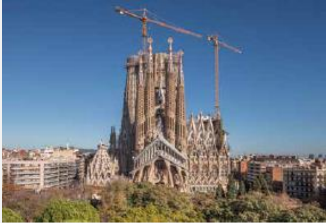
Fig. 2: The Passion façade features two 112 m (367 ft) bell towers flanked by two 102 m (334 ft) bell towers. Behind these, six more towers are under construction (© Fundació Junta Constructora del Temple de la Sagrada Família)
