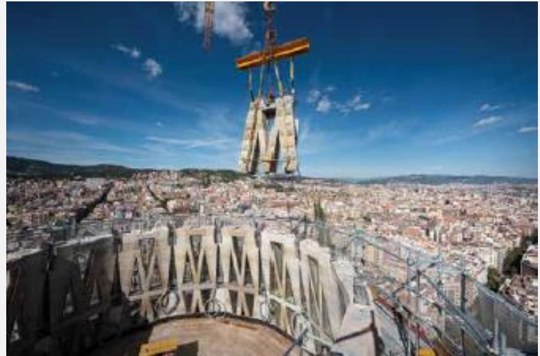
Fig. 7: Construction of central towers using prestressed stone panels reinforced by stainless steel columns joined with high-strength concrete (© Fundació Junta Constructora del Temple de la Sagrada Família)
