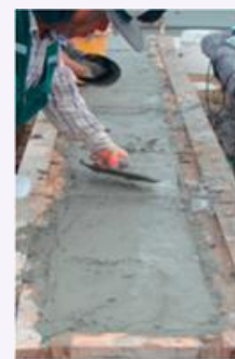
Figure 4: ECC reinforcement [16]
