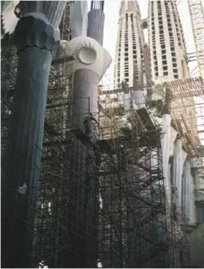
Fig. 6: Stone or precast concrete exterior “drums” were used to form the trunks and branches with reinforced concrete cores (© Fundació Junta Constructora del Temple de la Sagrada Família)
