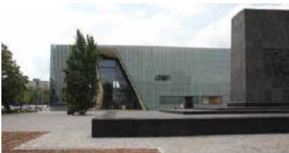
Fig. 1: The Museum of the History of Polish Jews in Warsaw, Poland. The museum stands in what was once the heart of Jewish Warsaw—an area which the Nazis turned into the Warsaw Ghetto during World War II. The building's simple form is split by a wide fracture directly opposite the nearby Monument to the Ghetto Heroes
