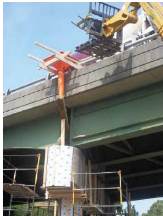
Fig. 4: SCC placed using a funnel and a chute
