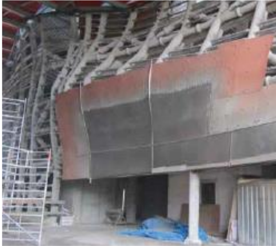
Fig. 9: After plywood panels were installed as stay-in-place formwork defining the wall curvature, anchors and welded wire reinforcement were installed, polymer strips were set to form expansion joints and to serve as depth guides, and the first layer of shotcrete was applied
