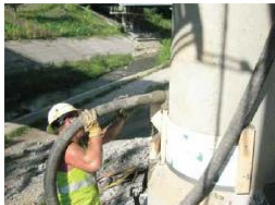
Fig. 5: SCC pumped into formwork
