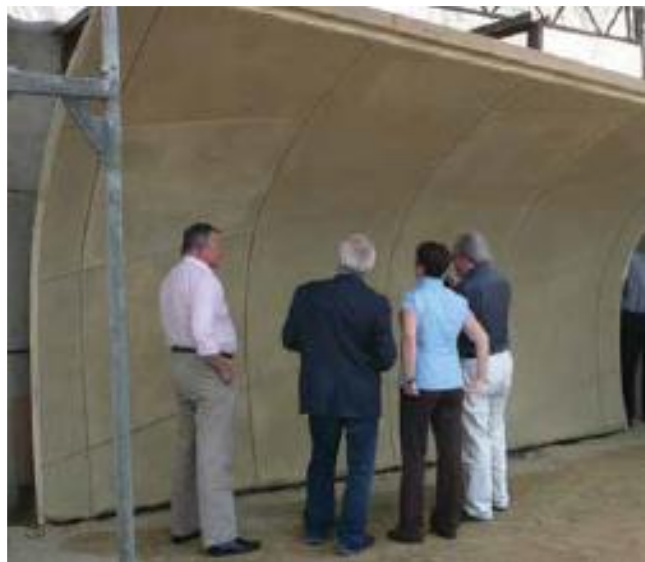
Fig. 4: Mockup of curvilinear wall divided into diamond-shaped elements. One of the designers, Rainer Mahlamäki, is on the far right
