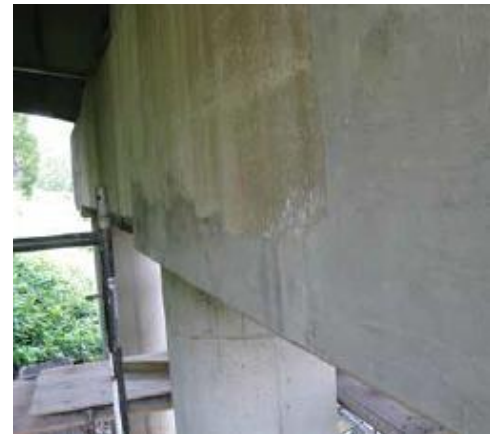
Fig. 7: Final state of the repair on the Route 712 bridge substructure
