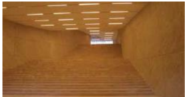
Fig. 2: The connecting tunnel from the second part of the building, the services compound, which consists of a single underground floor
