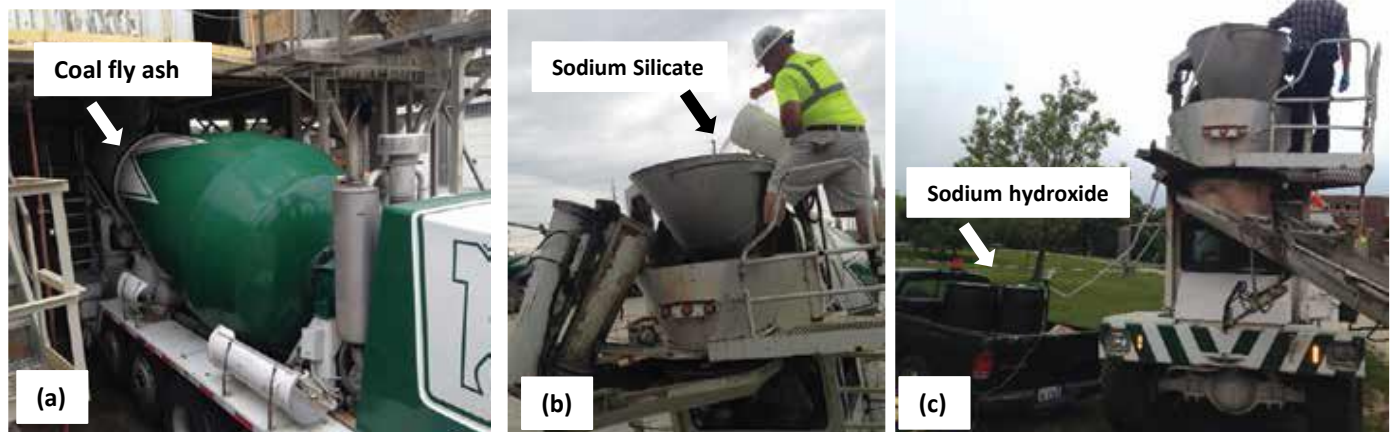
Fig. 4: Field trial of geopolymer concrete: (a) loading coal fly ash to a concrete truck; (b) adding sodium silicate solution at the plant; and (c) pumping sodium hydroxide solution into a mixer at the jobsite
