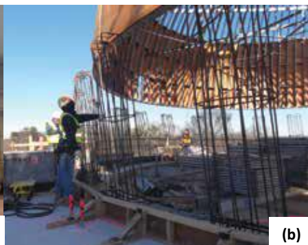
Fig. 9: The primary dome on the mosque was too large to be formed using EPS foam, so custom formwork was fabricated from crimped cold-formed steel shapes and plywood sheathing: (a) the Radius Track cold-formed shapes were assembled at the ground level; (b) the partially completed assembly was installed using a tower crane; and (c) the remainder of the dome formwork sheathing was fastened to the framing and the window formwork was installed (photos courtesy of Facchina Construction Company, Inc.)
