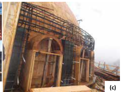
Fig. 9: The primary dome on the mosque was too large to be formed using EPS foam, so custom formwork was fabricated from crimped cold-formed steel shapes and plywood sheathing: (a) the Radius Track cold-formed shapes were assembled at the ground level; (b) the partially completed assembly was installed using a tower crane; and (c) the remainder of the dome formwork sheathing was fastened to the framing and the window formwork was installed (photos courtesy of Facchina Construction Company, Inc.)
