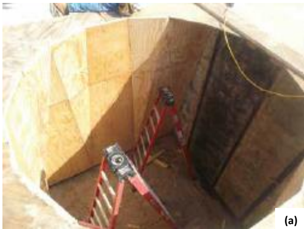
Fig. 11: The minarets comprise rectangular bases and polygonal towers: (a) the transition between base and tower was formed using dimension lumber and plywood sheathing; and (b) the tower was formed using a hybrid system comprising MevaLite wall formwork, dimension lumber, and plywood sheathing lifted into place using the site's tower crane (photo courtesy of Mostafa Fahimi, EyeConstruction, Inc.)
