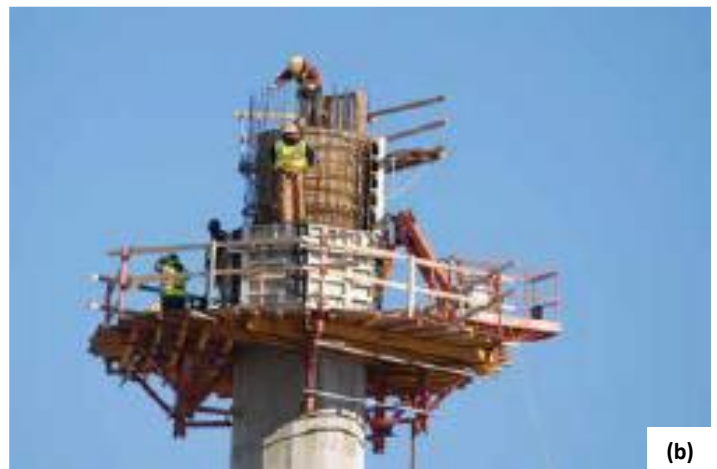
Fig. 11: The minarets comprise rectangular bases and polygonal towers: (a) the transition between base and tower was formed using dimension lumber and plywood sheathing; and (b) the tower was formed using a hybrid system comprising MevaLite wall formwork, dimension lumber, and plywood sheathing lifted into place using the site's tower crane (photo courtesy of Mostafa Fahimi, EyeConstruction, Inc.)
