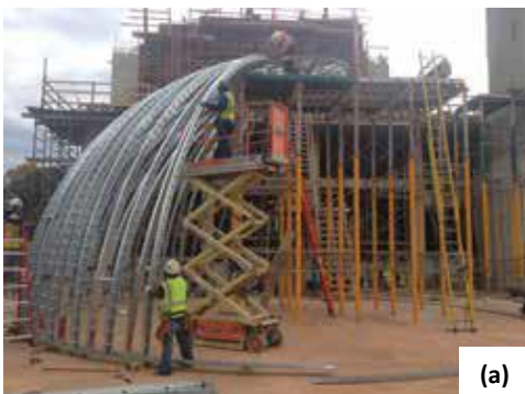
Fig. 9: The primary dome on the mosque was too large to be formed using EPS foam, so custom formwork was fabricated from crimped cold-formed steel shapes and plywood sheathing: (a) the Radius Track cold-formed shapes were assembled at the ground level; (b) the partially completed assembly was installed using a tower crane; and (c) the remainder of the dome formwork sheathing was fastened to the framing and the window formwork was installed (photos courtesy of Facchina Construction Company, Inc.)
