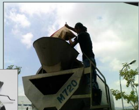
Photo 11: Steel fibre dispensing into concrete truck
