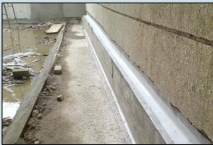
Photo 15: Hypalon Sheet for Bandaging Joints
