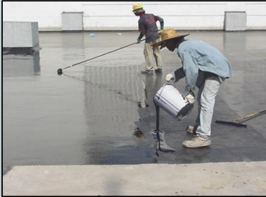
Photo 5: Liquid applied membrane (LAM)
