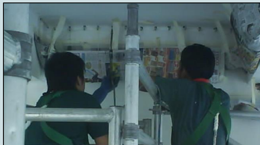
Photo 12: Pressure Grouting Polyurethane Grout
