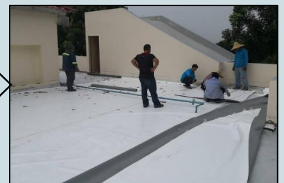
Photo 10: Preform TPO Membrane
