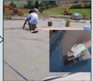
Photo 6: Reinforced Flexible Cementitious
