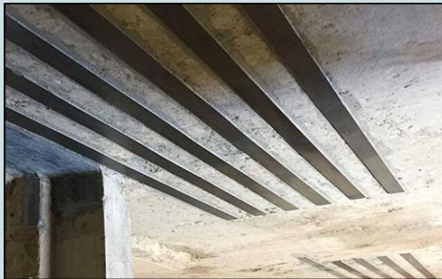
Photo 13: Carbon Fibre Plates for Strengthening of Concrete Slab
