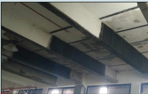
Photo 14: Carbon Fibre Fabrics for Strengthening of Concrete Beams
