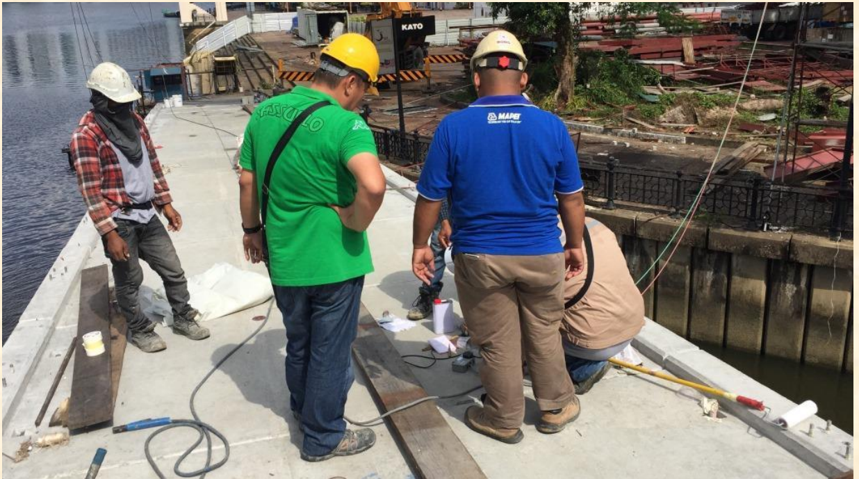
Checking substrate conditions
