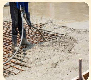
Vibration of Concrete
