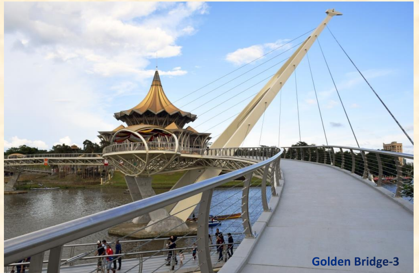
Completed coating works on the bridge deck
