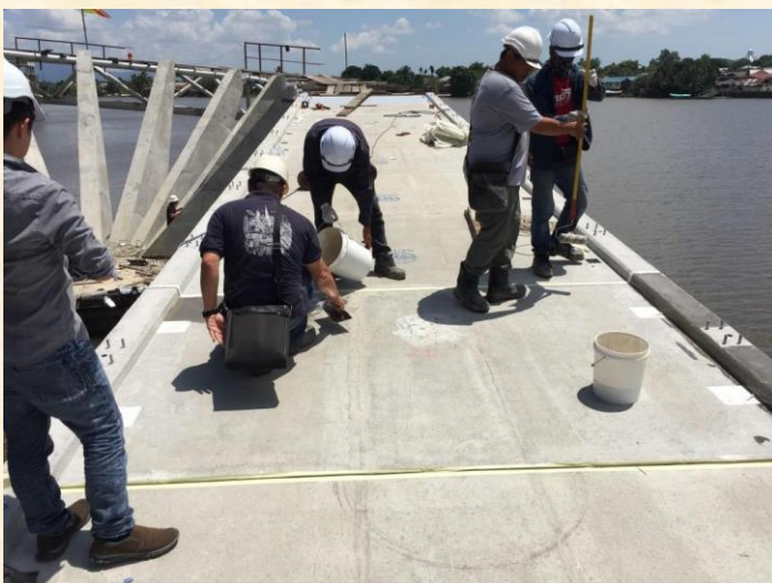
Getting ready to apply Primer SN on the concrete bridge deck
