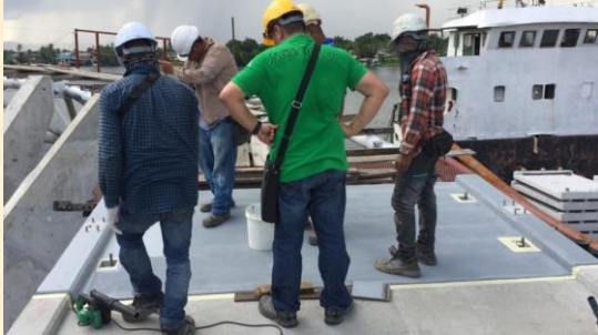
Application of the second coat of Mapecoat CF-AP
