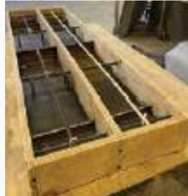
Fig. 6: Formwork, reinforcing bars, and crack initiator for shrinkage cracking test specimen preparation
