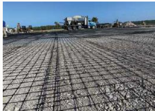
Fig. 5: FRP meshes can be used as secondary reinforcement in slabs-on-ground
