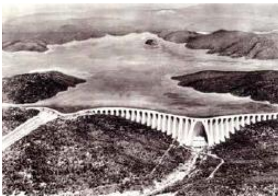
Fig. 3: Artist’s rendering of Andre Coyne’s multiple arch concrete dam design for the Oroville site (based on Reference 10)
