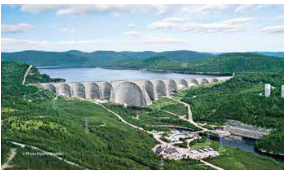
Fig. 2: Daniel-Johnson Dam and Manic-5 Generating Station in Quebec, Canada (photo courtesy of Hydro Québec)
