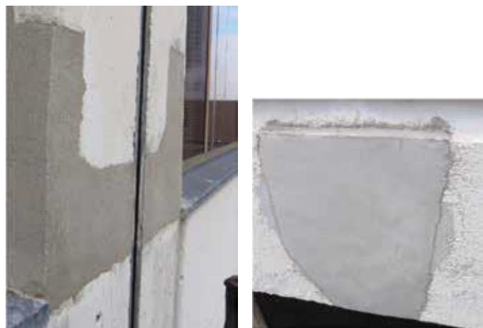
Fig. 8: Restoration of a 40-story reinforced concrete building in Philadelphia, PA, USA, in 2016. Spalled areas were repaired with a rubber-modified repair material. Repairs were to be subsequently covered with a polymer coating
