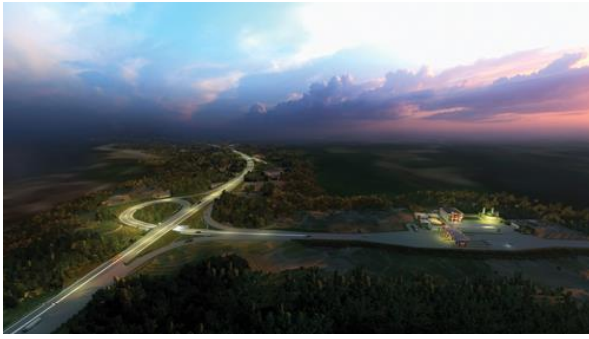
Trans Sumatera Toll Road Project Section Serbelawan-Pematangsiantar (image courtesy of PT Hutama Karya [Persero])
