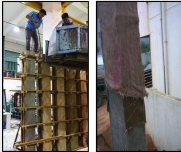
Fig. 4. Casting of column (left) and curing using gunnysack (right)
