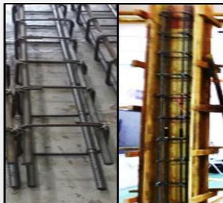
Fig. 3. Steel cage (left) and Formwork (right)
