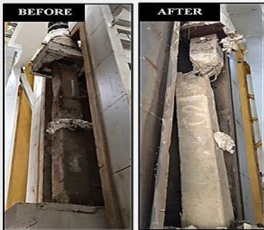
Fig. 6. Column before and after ASTM E119 fire test
