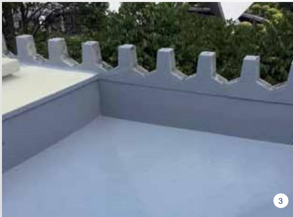
PHOTO 1. The frames embedded between the pyramids and the cupolas were first cleaned by hydroblasting. PHOTO 2. The substrates of the cupolas were waterproofed with PURTOP 1000. PHOTO 3. To provide further protection, the frames were treated with MAPECOAT PU 15 finish. PHOTO 4. The mosaic tiles were bonded to the cupolas with KERAPOXY and joints were grouted with KERACOLOR FF + FUGOLASTIC
